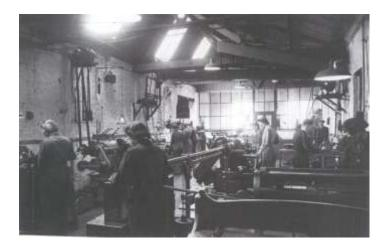
Centre lathes, capstan lathes and sheet metal guillotines
